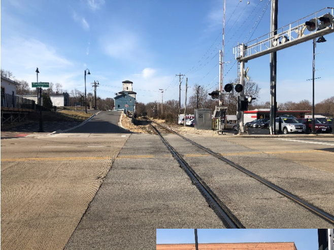
There is a railroad line that runs just west of Main St and is situated at the lowest point in the area, making significant modification of the grade cost prohibitive. In the picture below, the base of a crossing gate was placed in the middle of the sidewalk, creating a challenge to providing minimum sidewalk width.
